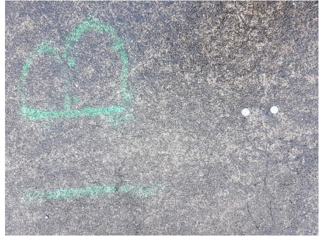
2. Level 2, 1B location.
