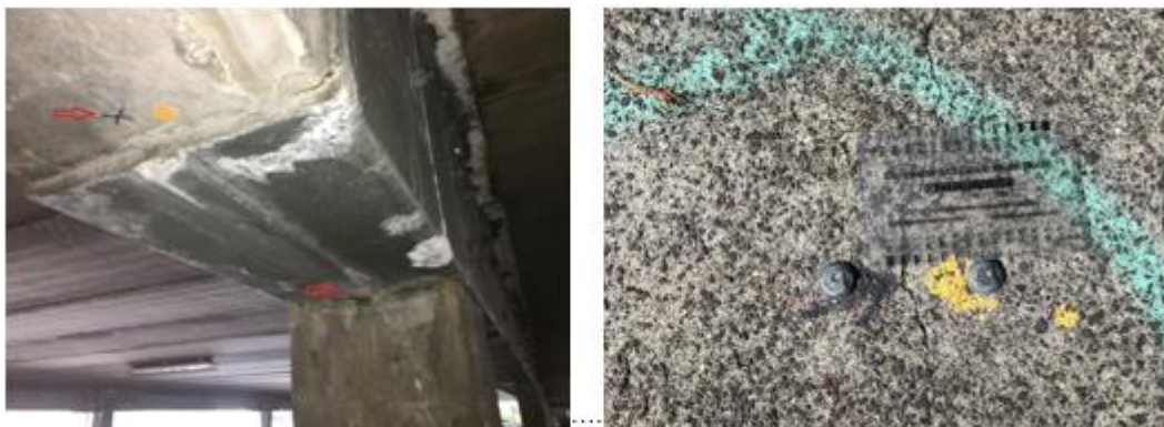
Figure 2: GHD deflection marking at IB2, IB3 and monitoring pins installed
